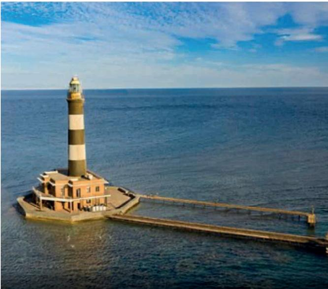
*TOP LEFT AND CENTRE: Ashrafi Reef was also called Ushruffee. It is located on a coral reef 54 miles south of Ras el Gharib where the channel into the Gulf of Suez is only 6 miles wide. The metal framework structure was replaced in 1940, but the original still exists nearby. The new tower is 140 ft high and the light was a white revolving light seen at 17 miles distant.*
